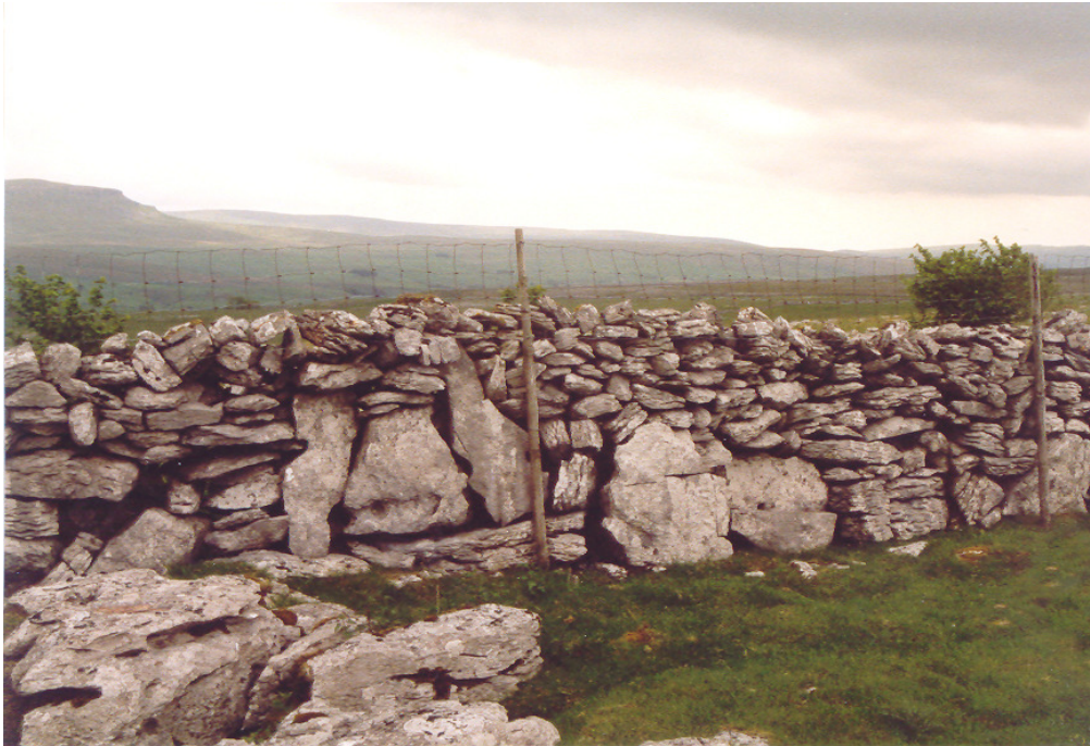
Plate 14 Three-quarter double wall with a row of upended limestone pavement orthostats. Fell Close boundary, Selside Upper Ribblesdale. The original topstones are missing, and the upper part of the wall has been modified by later repair. The wall is now stock proofed with galvanized top wire mesh fencing. When first built projecting topstones served as a deterrent against animals jumping from the fell. For the original profile on the fell side see Plate 11.
