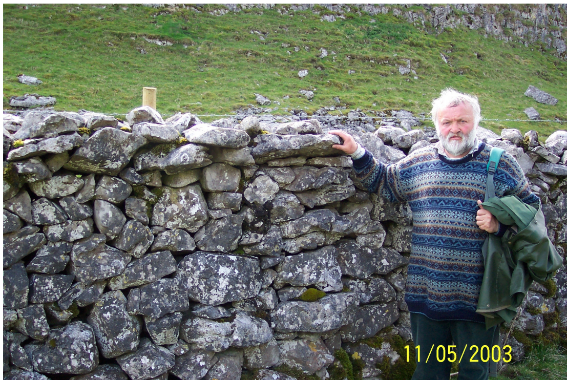
Plate 3 A wide top double wall with projecting topstones, Watlowes, Malham. This was part of the mediaeval boundary dividing the Malham outfield. Here the projecting topstones provide an additional deterrent against animals jumping into the Fountains Abbey side, on the other side of the wall.
