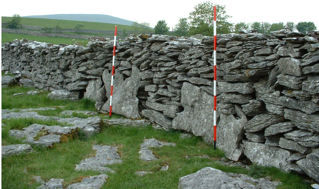
Plate 4 A well preserved wide top double wall with projecting topstones and orthostats at the base of the wall. The limestone bedrock provides a stable foundation, and the survival of the original wall structure is excellent. Ingman Lodge boundary wall, Upper Ribblesdale.
