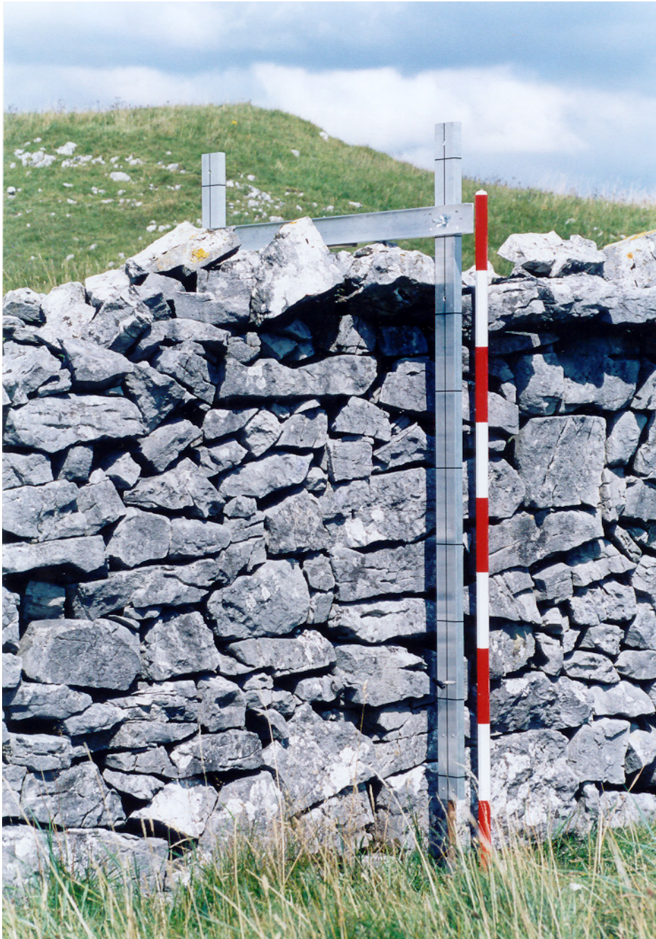
Plate 2 Another part of the Winskill infield boundary wall viewed from the outside. It is a wide top double wall with some of the original projecting topstones still in place. The projecting topstones provide an additional deterrent against animals jumping into the infield area. The wall is built here almost directly on limestone bedrock.
