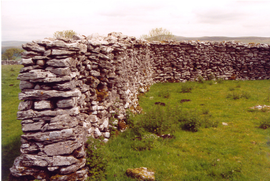
Plate 9 Wide top double wall head with projecting topstones facing into the gathering pen in the Furness Abbey 'bercaria' complex at Selside (Fig. 2 & Plate 9). The arrangement of the topstones may have been necessary to control sheep especially prone to jumping. Flocks of weathers, castrated male sheep kept for wool and meat, are a possibility.
