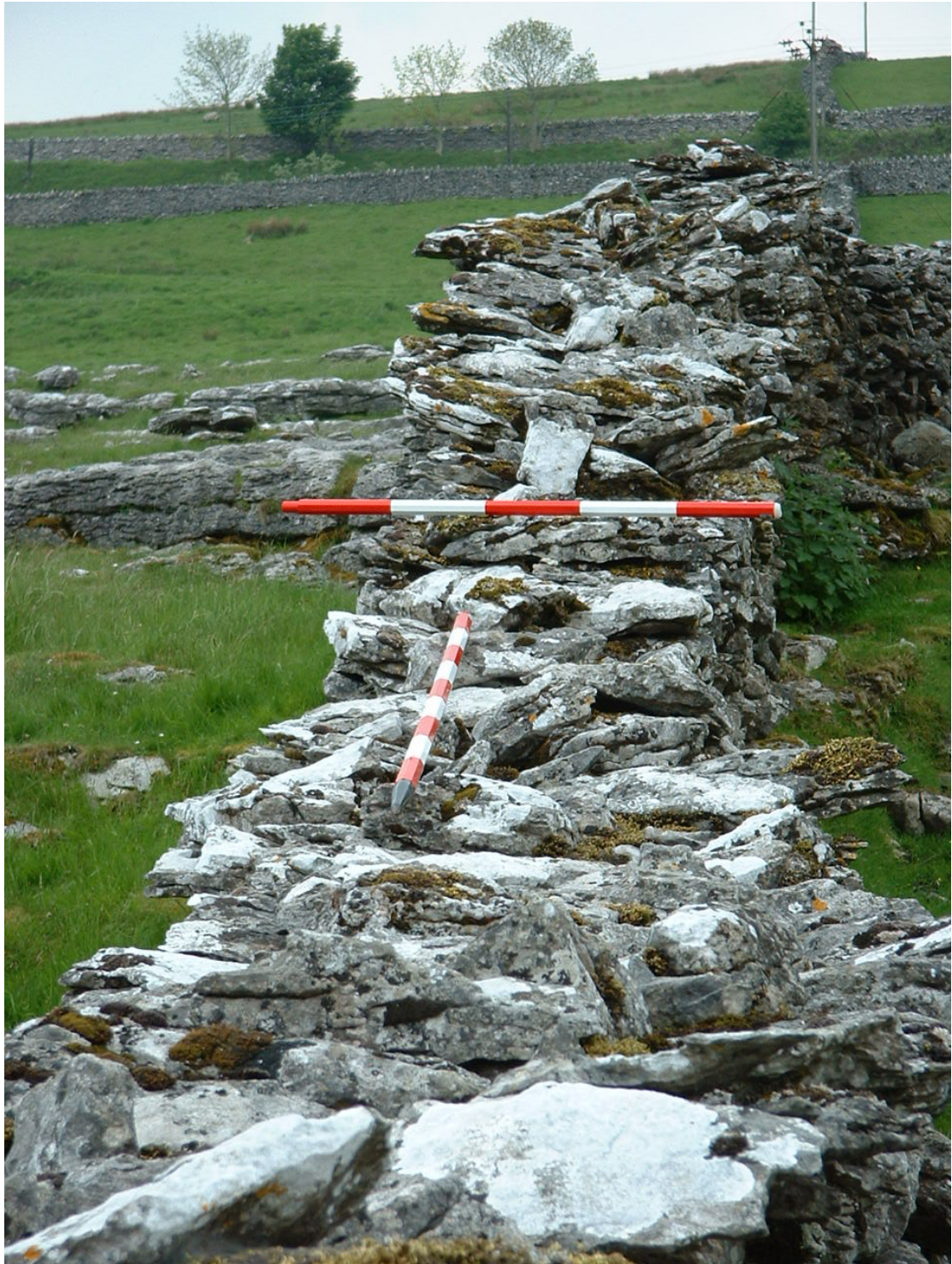
Plate 6 Wide top double wall with projecting topstones on both sides of the wall. Ingman Lodge boundary, Upper Ribblesdale. This wall stands around 1.6 metres high (about 5ft 4 inches). Like most wide top double walls the width of the top of the wall beneath the topstones is 50 cm (20 inches). The topstones project on each side about 15 cm (6inches). So far such topstones have been recorded only at Selside. They might be a design restricted to Furness Abbey holdings.
