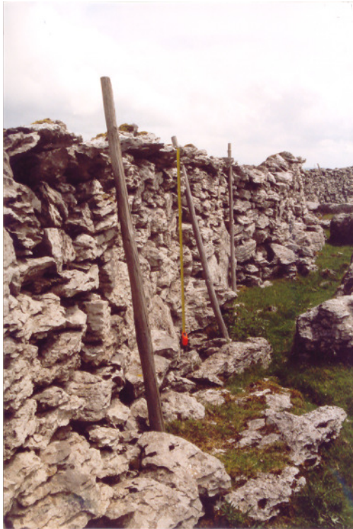
Plate 11 Three-quarter double wall made from weathered limestone, Fell Close boundary, Selside, Upper Ribblesdale. Tape 1.2 metres (4ft).
