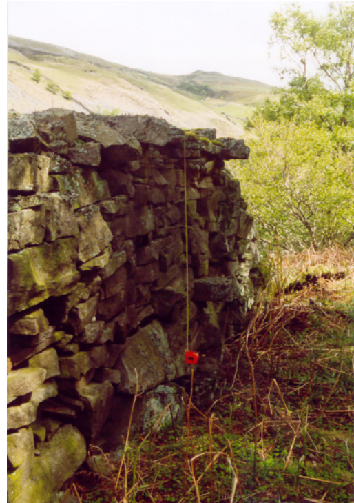
Plate 12 Three-quarter double wall made from field clearance sandstone Gunnerside Gill boundary, Swaledale. Tape 1.2 metres (4ft).
