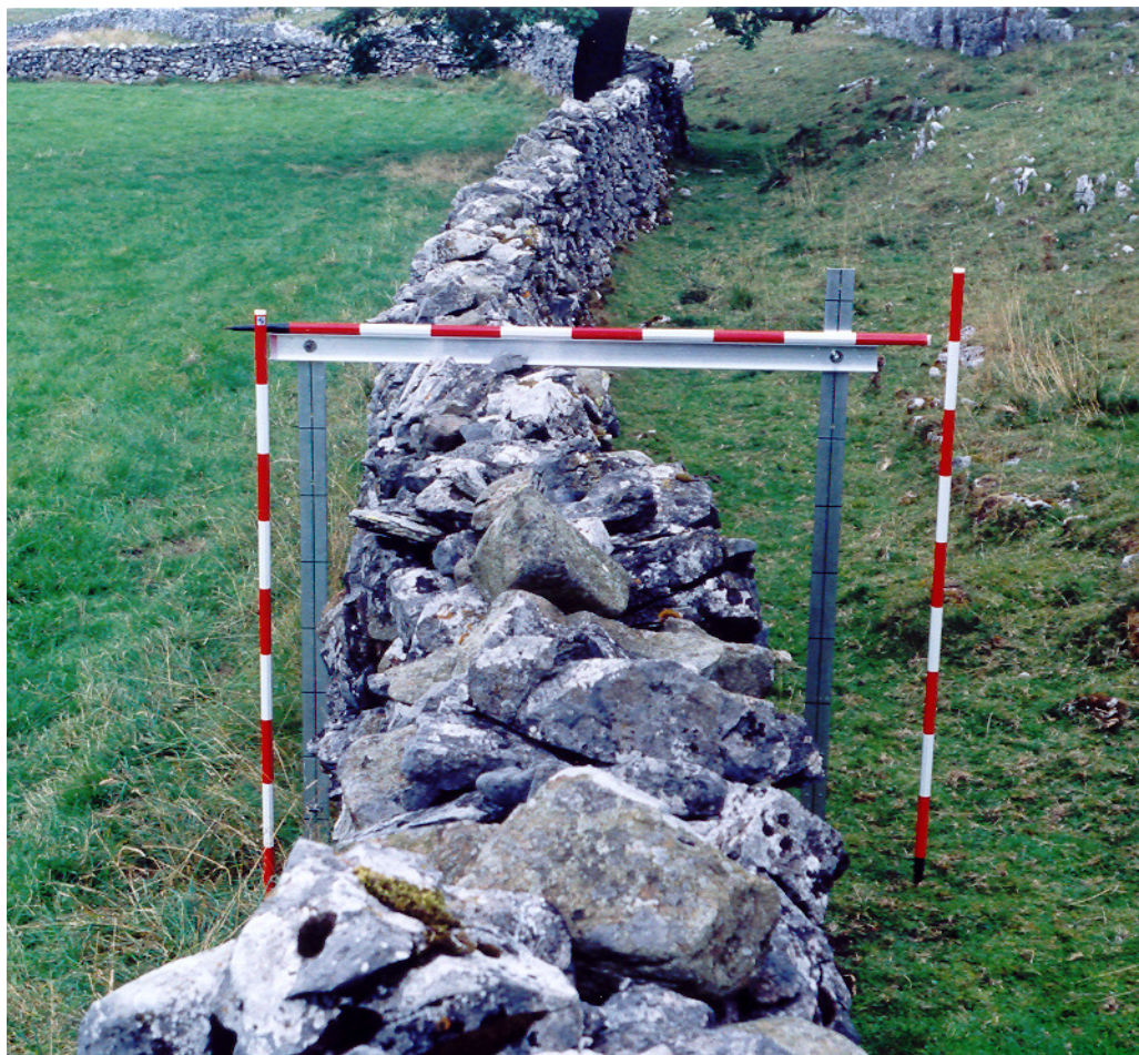
Plate 1 Documentary and field evidence indicates that this wall was standing in 1592. It was built earlier as part of the infield boundary at Winskill, Upper Ribblesdale. It is a wide top double wall and survives virtually as it was built apart from the loss of original topstones. The adjustable metal wall profile frame is an entirely new survey tool developed by the project to improve the recording of dry stone walls.
