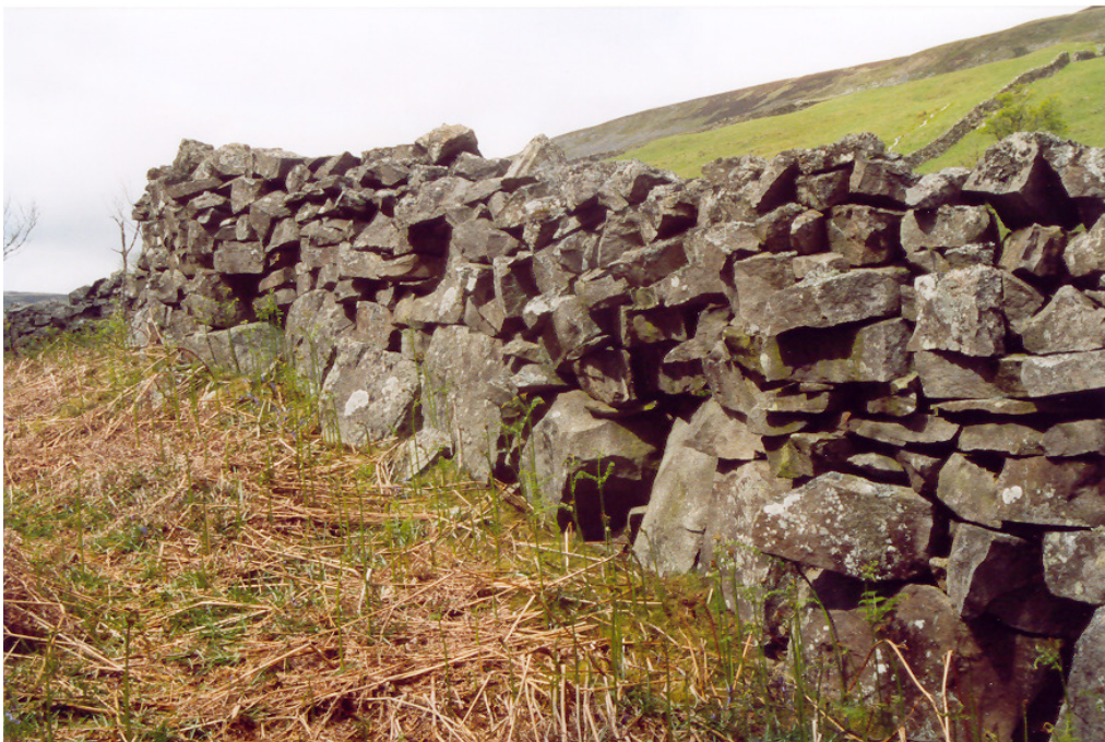
Plate 15 Three-quarter double wall with a row of blocky sandstone orthostats. Gunnerside Gill boundary wall, Swaledale. The wall is made of field clearance sandstones. The upper part of the wall has been modified by later repair. For the original wall profile on the gill side see Plate 12.
