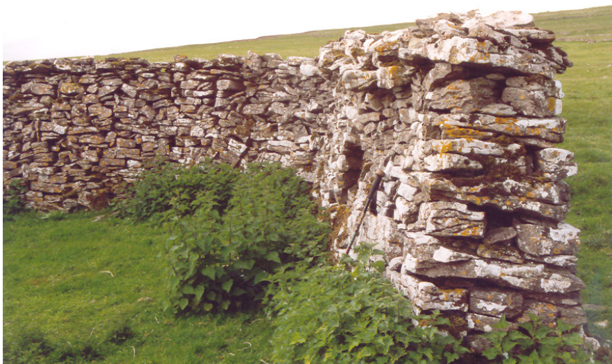
Plate 10 Wide top double wall head in the open D shaped fold in the Furness Abbey 'bercaria' complex at Selside. Note the projecting topstones facing into the fold area. This fold may have served a specialist function and would have required hurdles to stock proof the open side. It probably survived because it also served as a 'bield' or shelter wall for livestock, a purpose for which the inward facing projecting topstones are entirely unnecessary.
