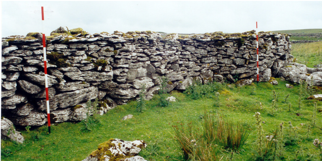
Plate 5 Wide top double wall with projecting topstones facing onto Borrins Moor, Selside, Upper Ribblesdale. The wall stands about 1.6 metres high (5 feet 4 inches).
